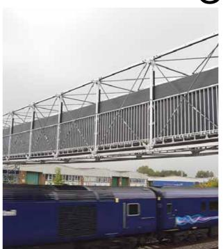
The versatile bridge system is designed to be used as a temporary public footbridge for projects involving temporary railway, road or river crossings - or to act as a beam structure to support other structures such as scaffolding or temporary roofs. The HBS may be constructed:
