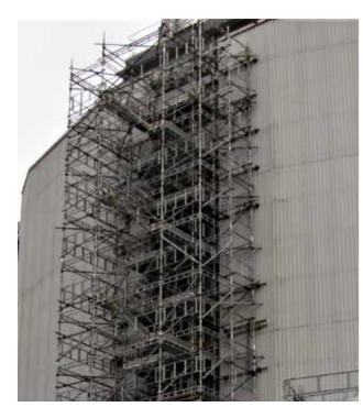
Stair towers provide a safe and quick access and egress to the workplace. The modular design and lighter components make the stairs quick and simple to erect.
